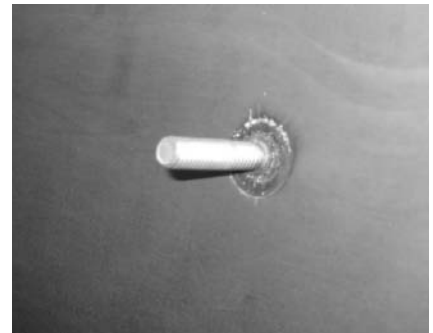
c.) Completed Stud
